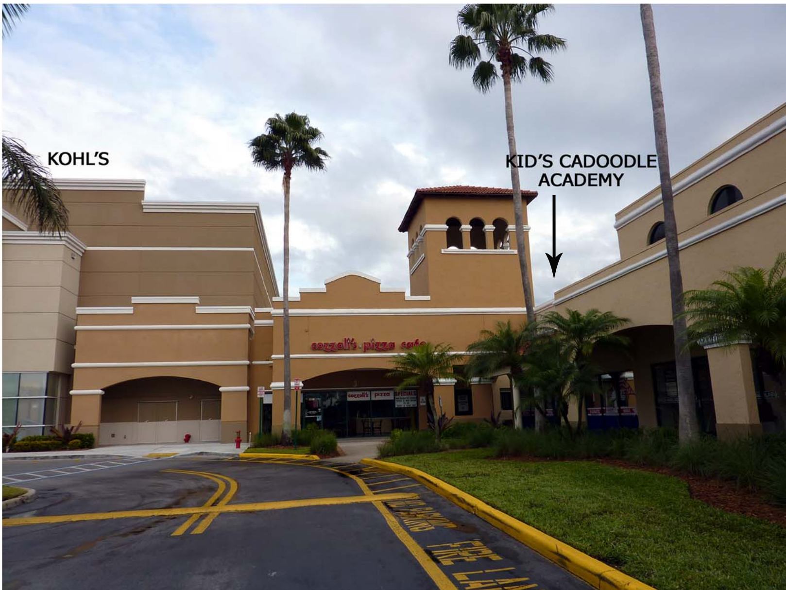
ADJACENT TENANTS: SOUTH FACADE
